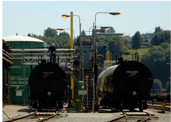
Above: One of our rail car loading areas on site
